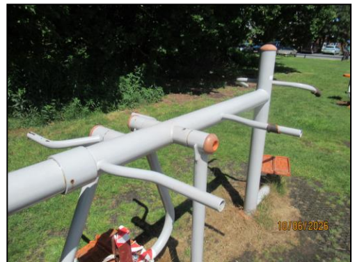
(Missing hand grips)
