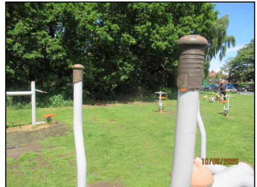
(Damaged hand grips)
