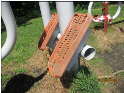
(Missing end cap at leg press)
